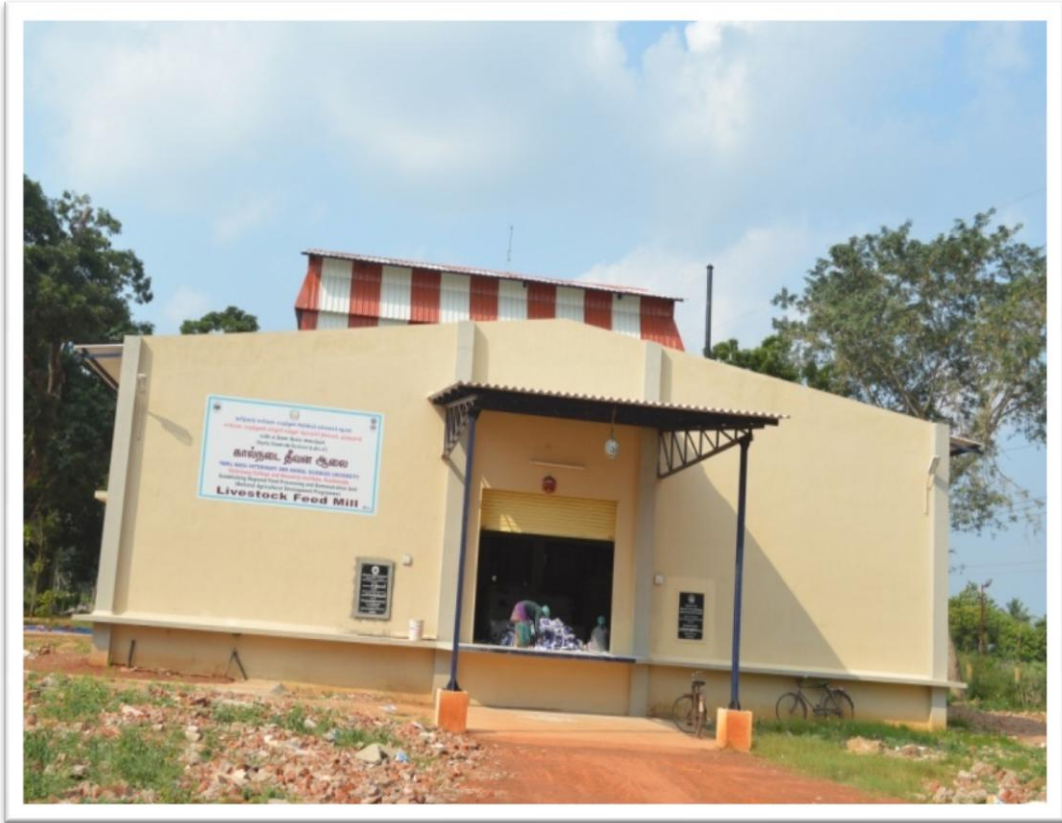
FEED PROCESSING UNIT
